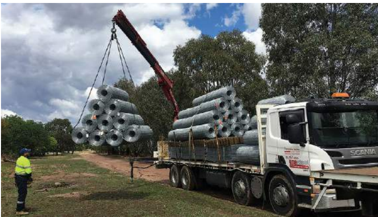
Fig 7.14: Unloading rolls of steel mesh shipped direct from the manufacturer to a central location.
