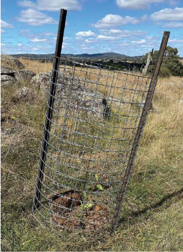
Fig 7.5: Tree guard installed at an angle with its bottom parallel to sloping ground to stop rabbits getting underneath.
