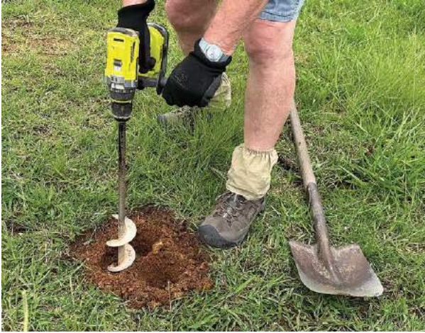
Fig 6.3: Using a drill and 600 mm long auger of 75 mm diameter to drill 3 holes for planting.
